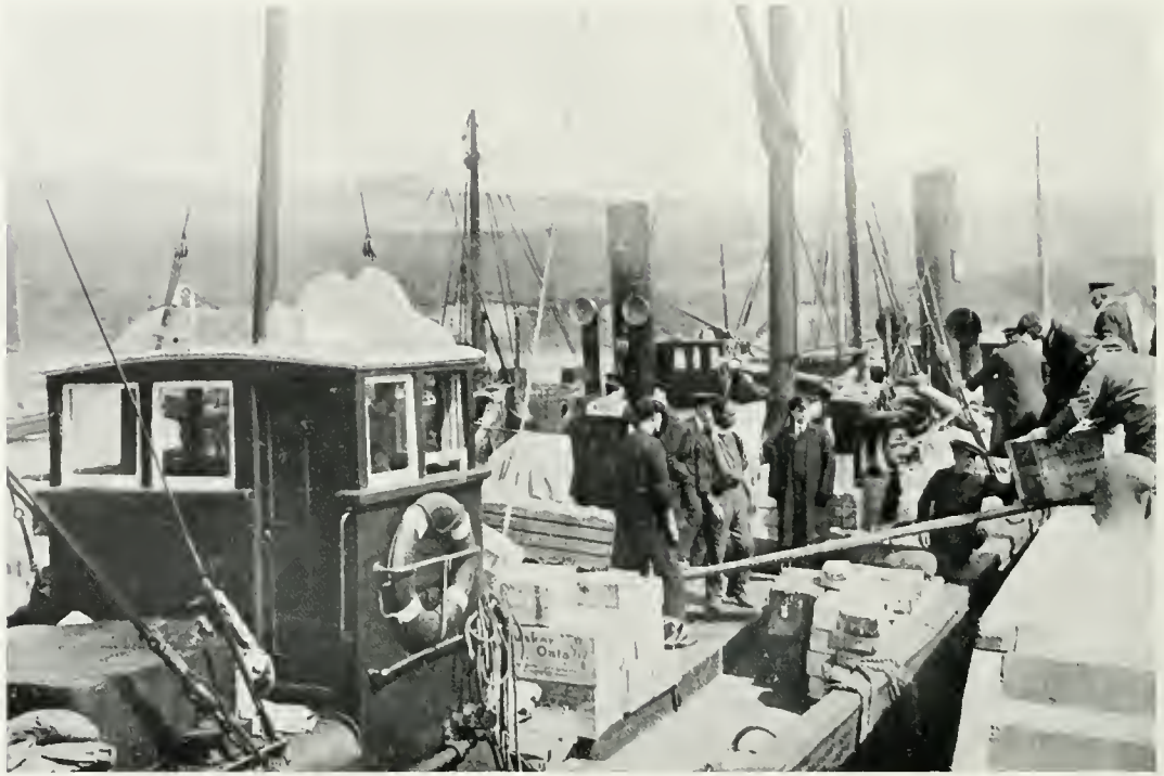
LOADING STORES AT SCAPA PIER.
